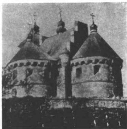
THE FORTIFIED CHURCH IN SUTKIVTSI—1476
