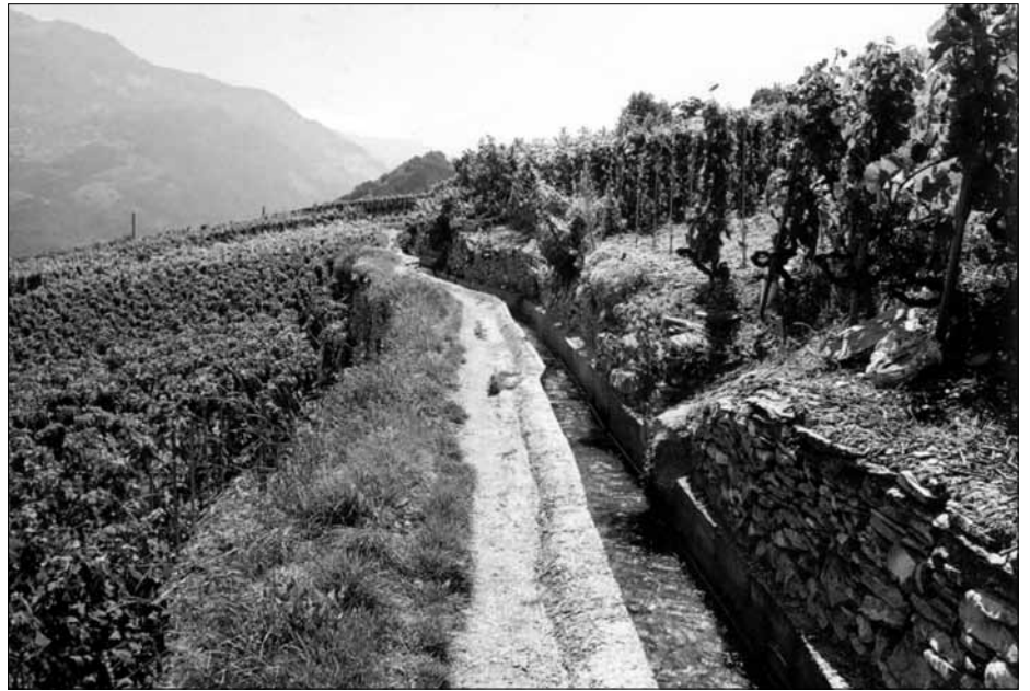
The Bisse de Sillonin near Saint-Léonard and the Bisse de Lentine near Sion still serve current water supplies for vineyards. (picture Giro Annen)
