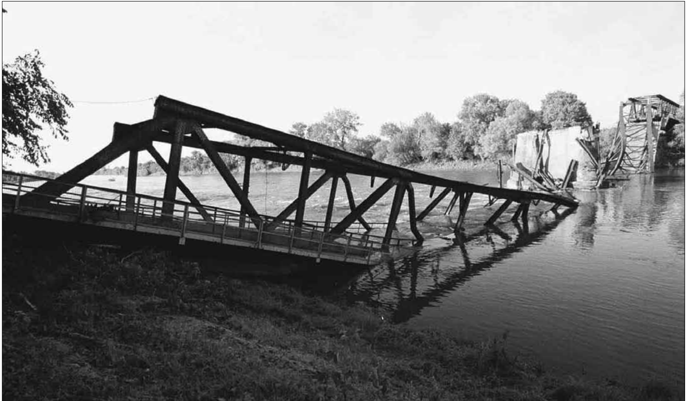
The bridge of Varvarin. (picture dpa)
