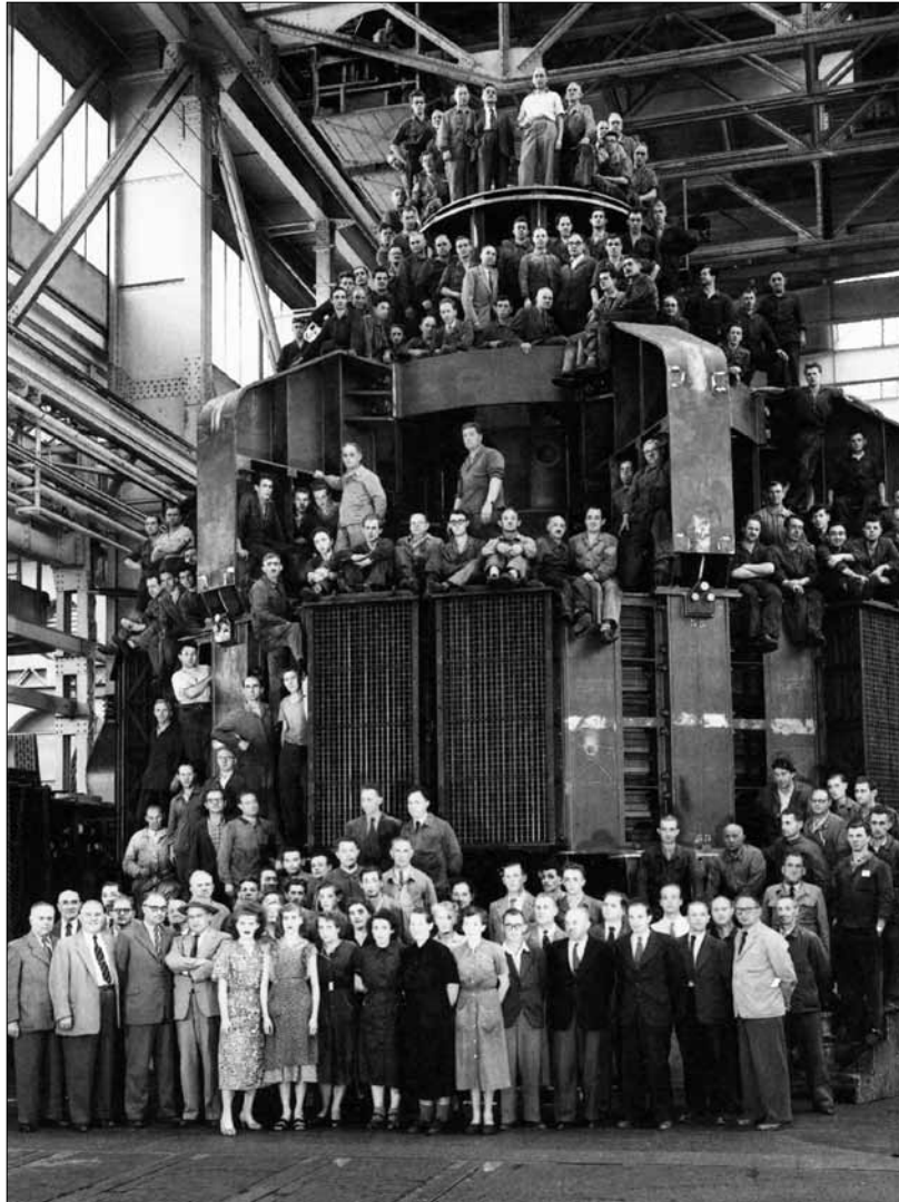
Hydroelectric generator for the Nile power plant Aswan, 1952, three groups of machines per 49,500 kVA by BBC, vertical axis, 100 U/min. (Picture Historical Archive ABB Switzerland)
