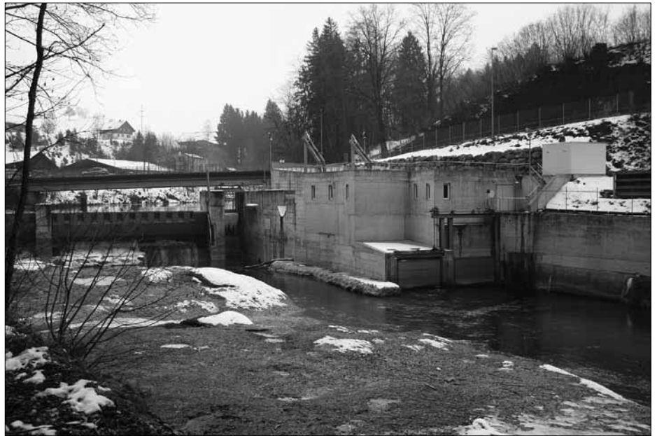
This small hydro power installation provides 1,300 households with electricity. (picture thk)
