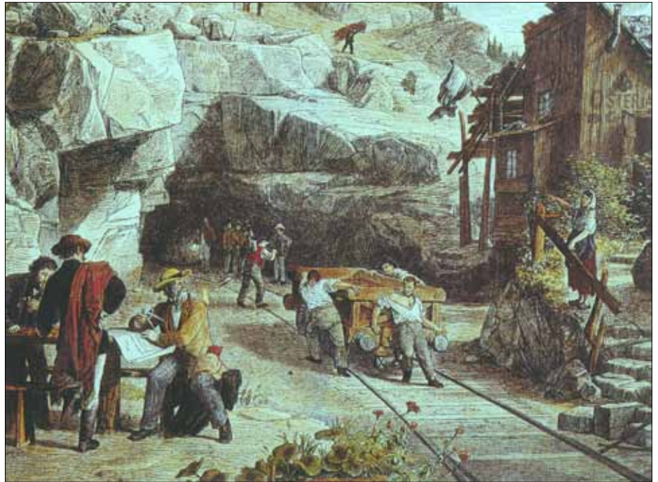
Scene at the south portal of the Gotthard tunnel during the construction works. (Picture exhibition Alfred Escher, catalogue ISBN 3-908225-08-6)
